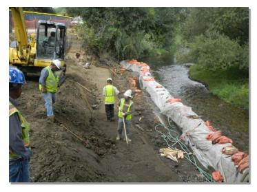
**Photograph TDM-1.** This coffer dam, installed to allow grading and stabilization of the stream bank, consists of concrete blocks covered by an impermeable linear held in place by sand bags.
